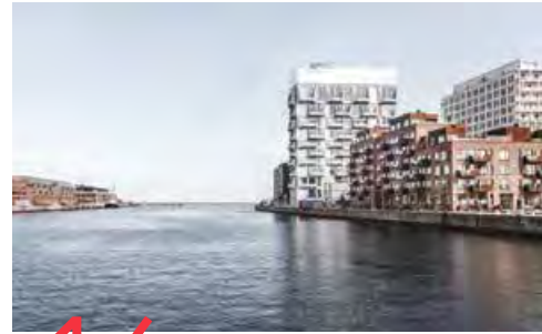
16 Silo in Copenhagen Microtopping®
